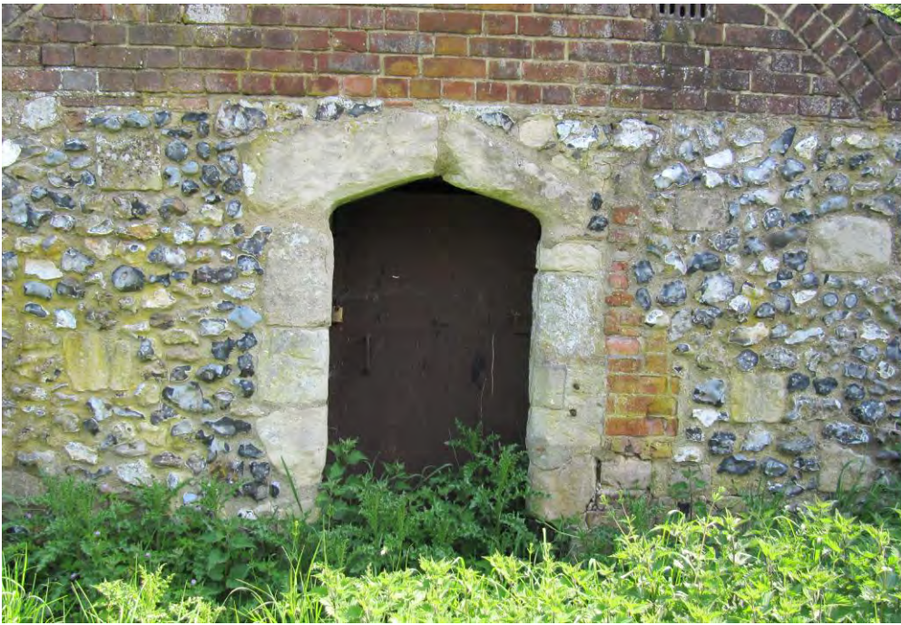
10 water source in Military Road
