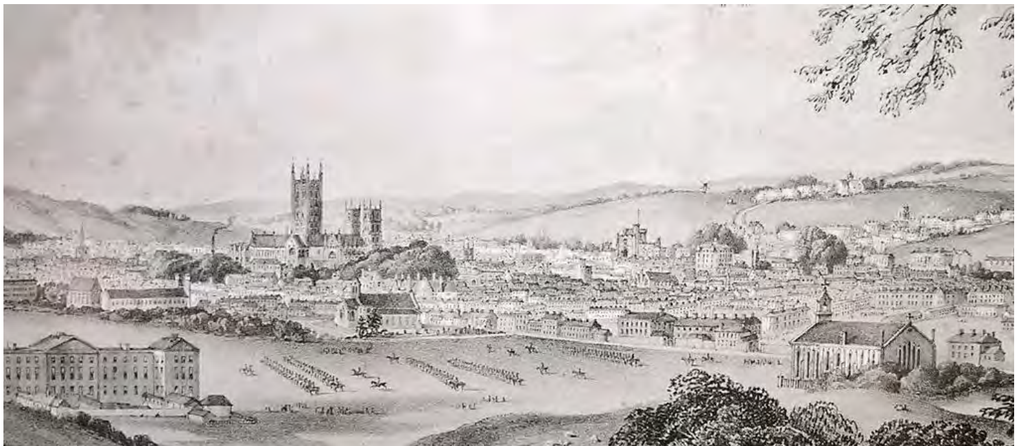
4 Westgate Museum (temporarily closed) - part of an early 19th century view of Canterbury including troops at Canterbury barracks
