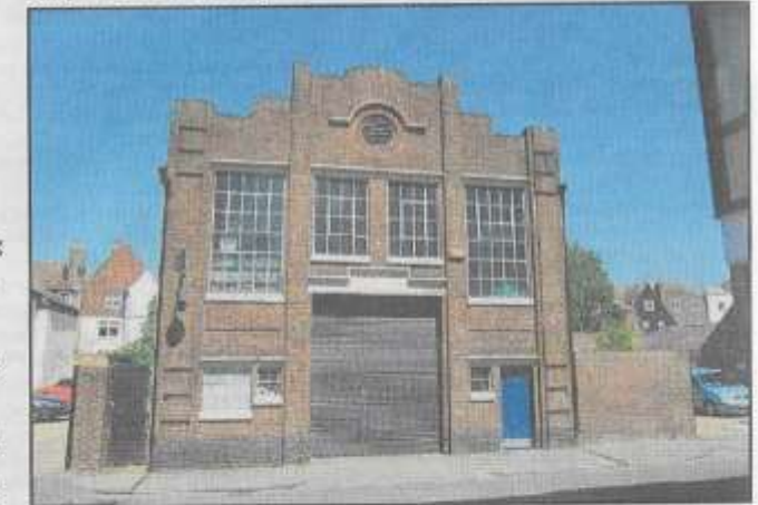
GRID: The old sub-station in Beer Cart Lane, now part of Furley Page Solicitors
