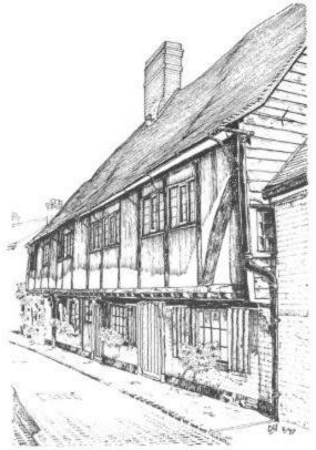
Il Saints Court dates from the fifteenth century and is a typical Kentish Merchants House. The main structure is a timber frame with the walls infilled between the timber structural members with wattle and daub, the wattle being a panel of woven split laths and the daub, a kind of plaster reinforced with animal hair and finished with a white limewash. The roof is steeply pitched and covered with small, hand made, clay tiles. Originally, the upper floor consisted of three chambers.
