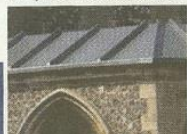
Typical DRYSEAL work on a grade I listed church.
