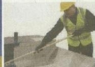
Standard DRYSEAL application procedure for flat roofs.
