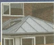
New conservatory with DRYSEAL roof. Traditional lead look to satisfy planning requirements.
