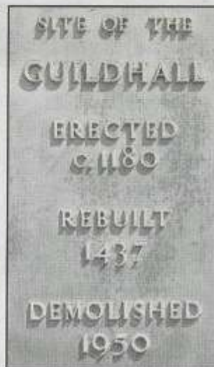
SIGN OF THE TIMES: All that's left of the Guildhall site
